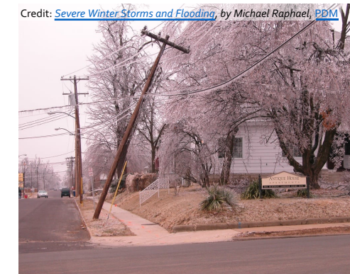
Fallen Power Lines
